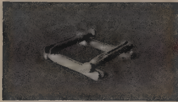
Fig. 2.—The block-house foundation,
